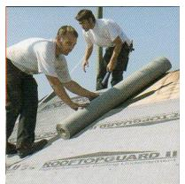
underlayment will be left exposed to the weather for an extended period of time, seal all seams with a butyl rubber, urethane, or EPDM based caulk or tape sealant.
